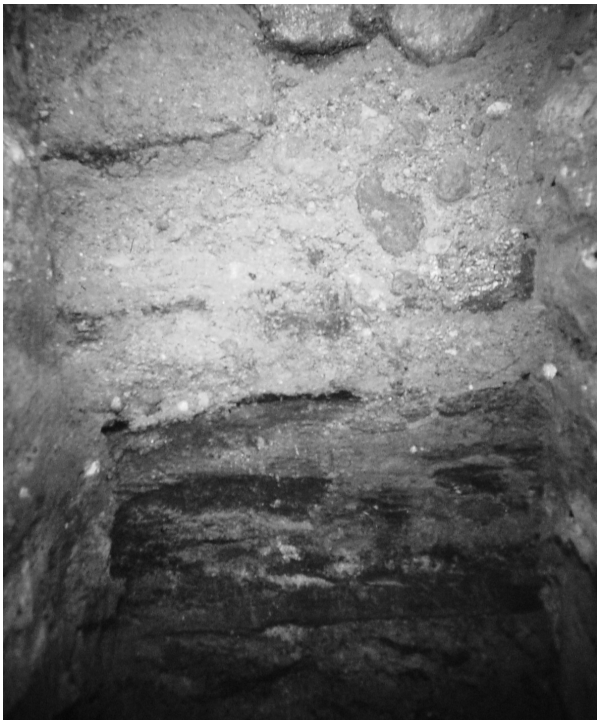
Fig. 3 Side view of excavated foundation wall (1995).
