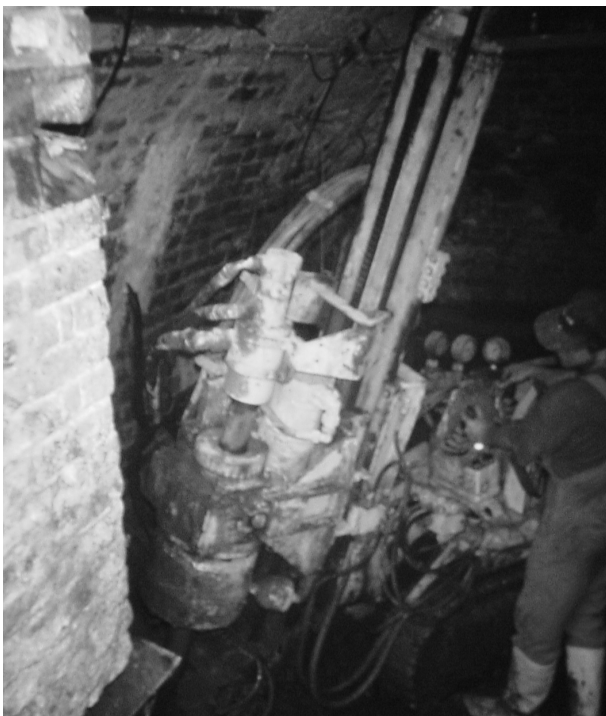
Fig. 10 Soilcrete works in a limited space in cellar
